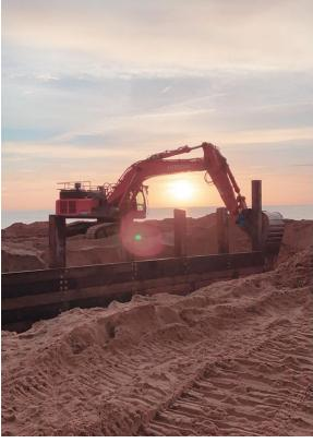
Installation of the piles commences nearest to the promenade, working towards the sea. Each pile location is marked using a robotic total station and steel pins, with protective caps. A leader mounted auger drills down to an agreed depth. To a high degree of accuracy, piles are driven with a Movax attachment mounted on a 35-tonne excavator. This process had been meticulously considered to avoid causing later deflection of the installed pile line.
